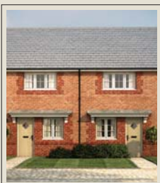
The above illustration is a typical example of a Broadway and Evesham.
