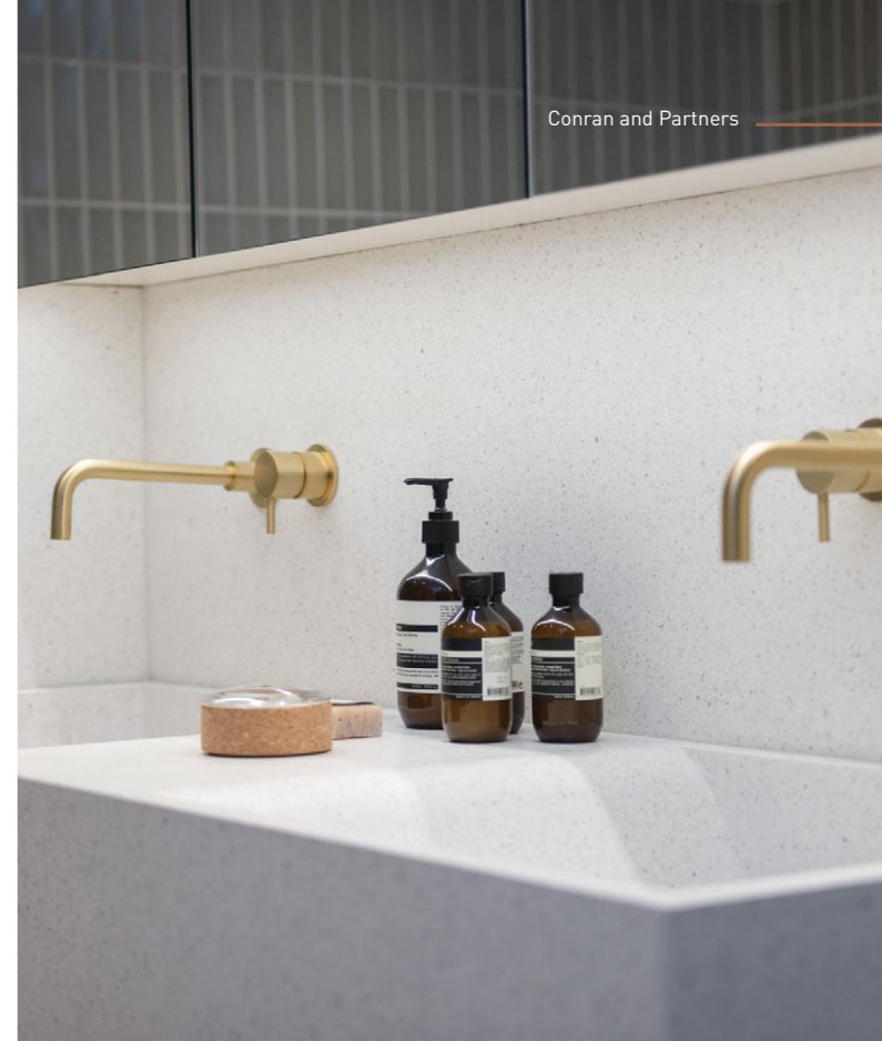
Using terrazzo sourced from Italy, the hand-carved vanity basins feature a hand-finished curve derived from forms found within the Barbican.
