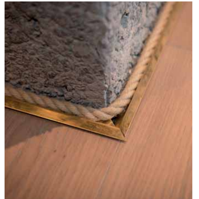
Many apartments benefit from exposed original concrete walls, with a rope junction between the concrete and the timber flooring.
